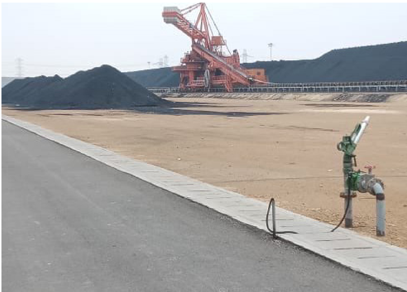
Coal storage at Jamshoro power plant
